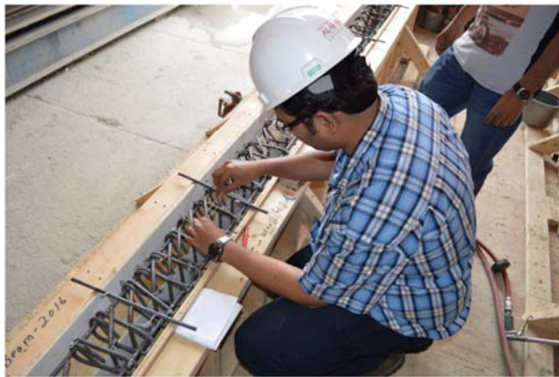
c) Students installing the concrete strain gauges
