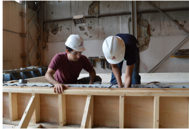
b) Students inspecting the formwork preparation
