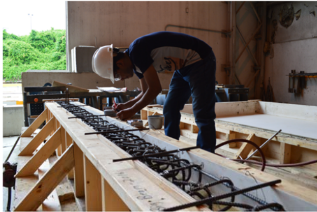
a) Formwork before casting
