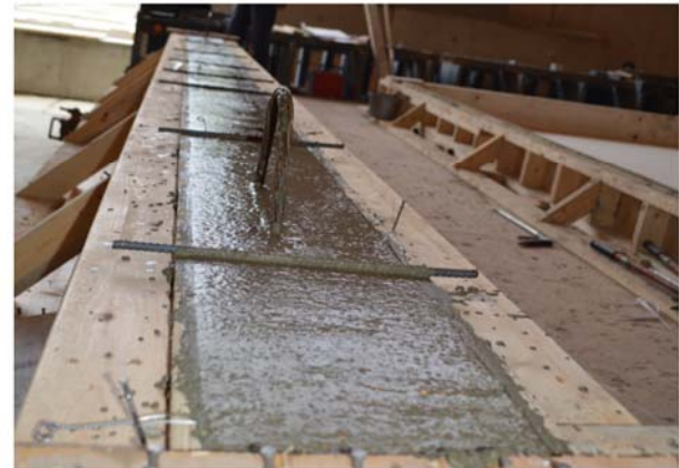
d) Finished Beam
