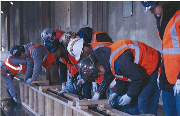
Figure 8: Inserting Prestressing Strands
