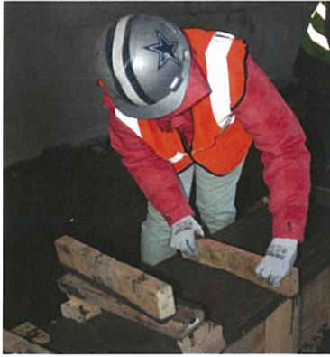
Figure 10: Concrete Finishing
