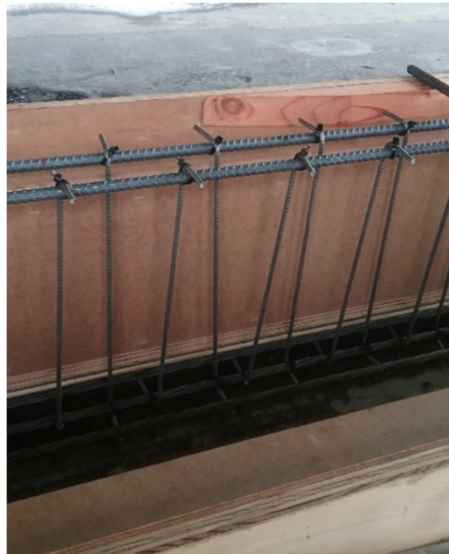
Figure 4: Stirrup Installation
