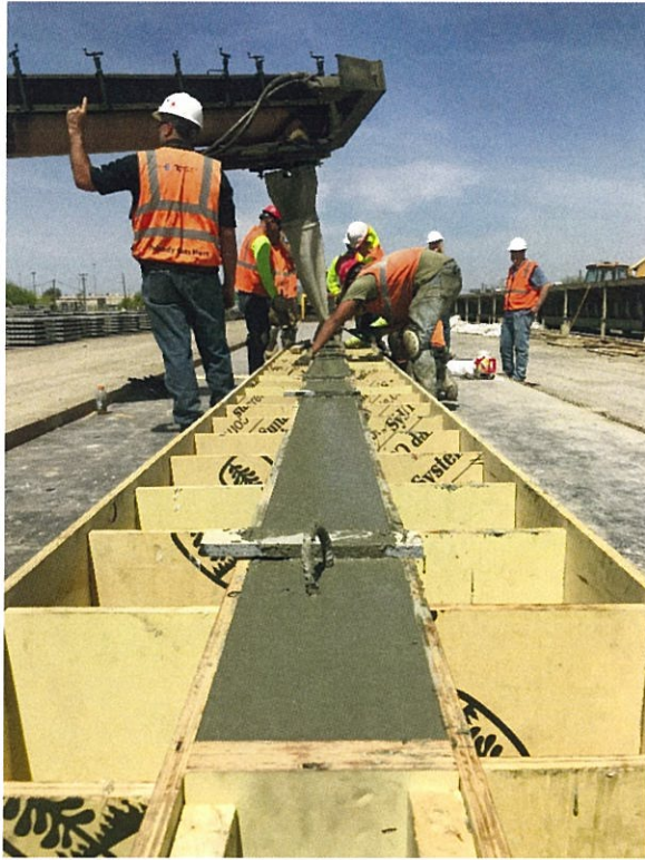
Figure A-5: Concrete Casting.
