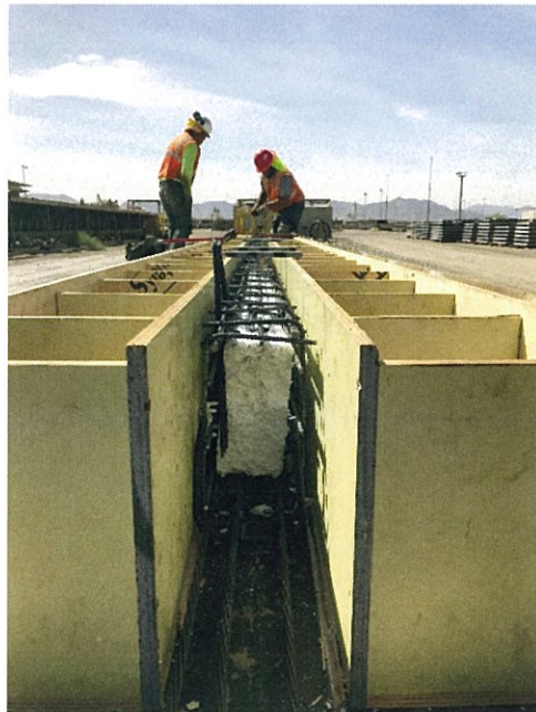
Figure A-4: Formwork – Side View.
