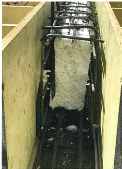
Figure 1: Formwork – Side View.
