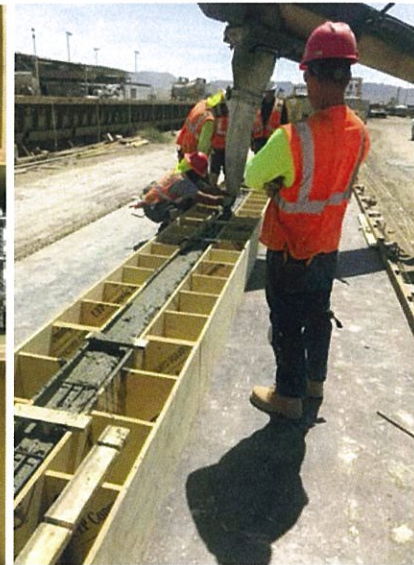
Figure 3: Beam Casting.
