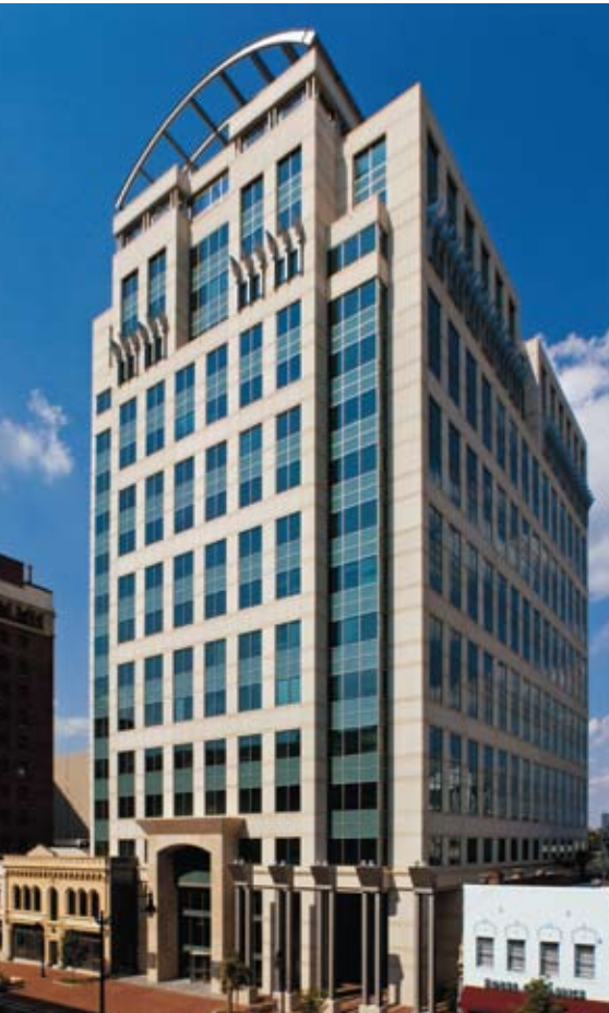
Meridian, Columbia, S.C.; Architect: SWSC; Photo: ©2003 Brian C. Robbins, Robbins Photography Inc.
